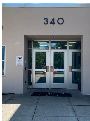
Kindergarten — Main Entrance
